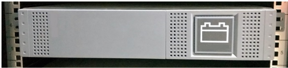
Figure 10.10. Rack-mountable uninterruptible power supply (UPS)
